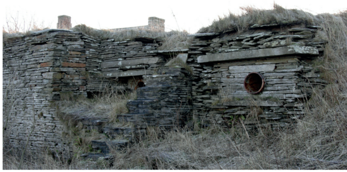
The sluices that fed the overshot wheel can still be seen today
